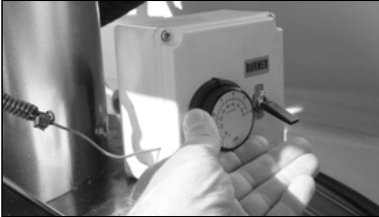
*Figure 5-53. Set the water heater thermostat.*
