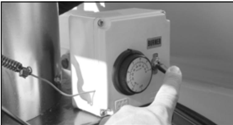
*Figure 5-54. Turn the water heater off by pressing the switch down.*
