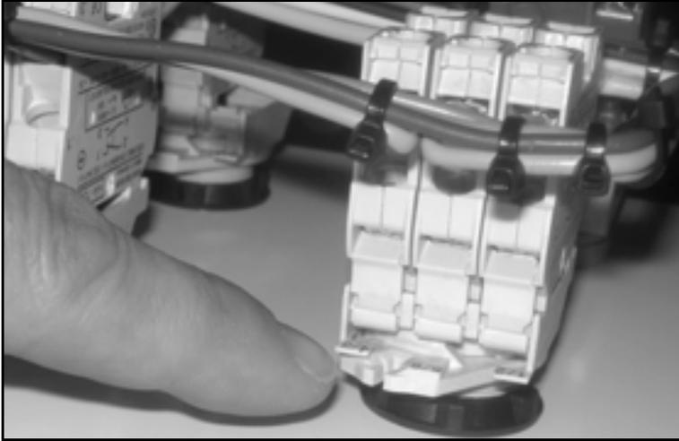
*Figure 7-11. The locking ring shown holds the body of the switch to the front section.*
