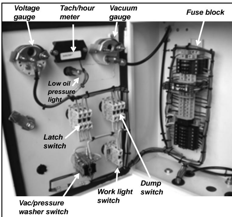
Figure 7-8. Control panel components and fuse block.
