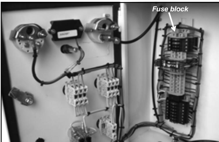
*Figure 7-15. Identify the blown fuse in the fuse block.*
